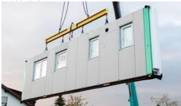
Figure 6 and 7: Transportation and movement of prefab elements/walls and materials
